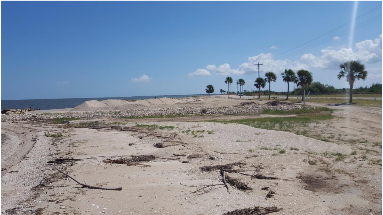
Southeast of STA 38+00
