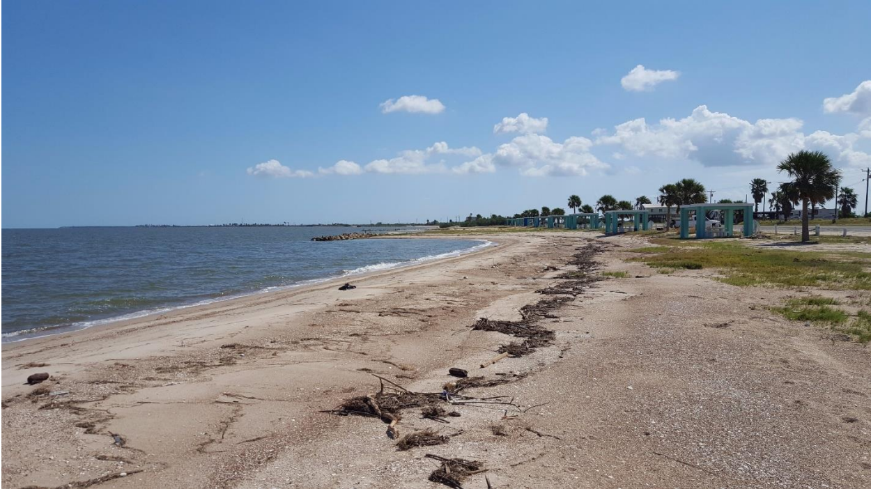
Southeast of STA 10+00
