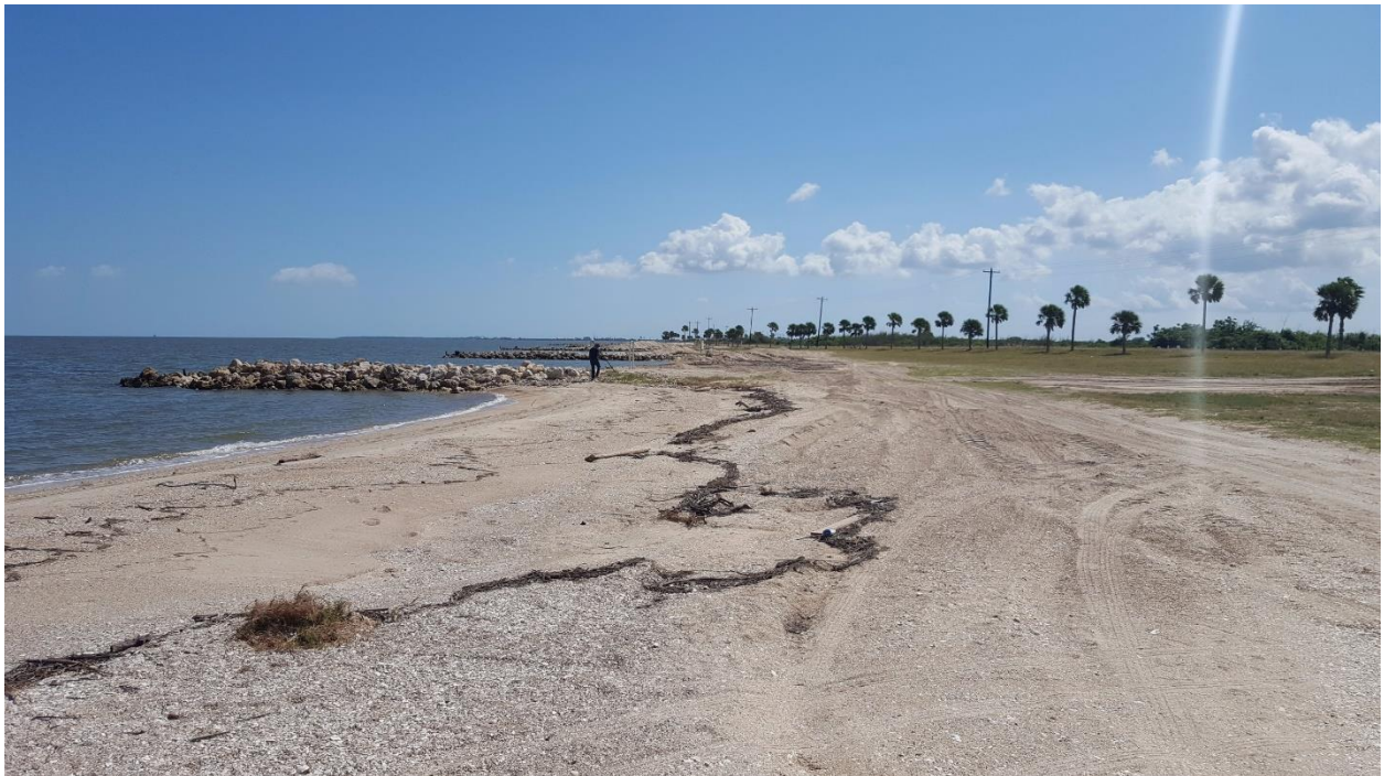
Southeast of STA 47+70
