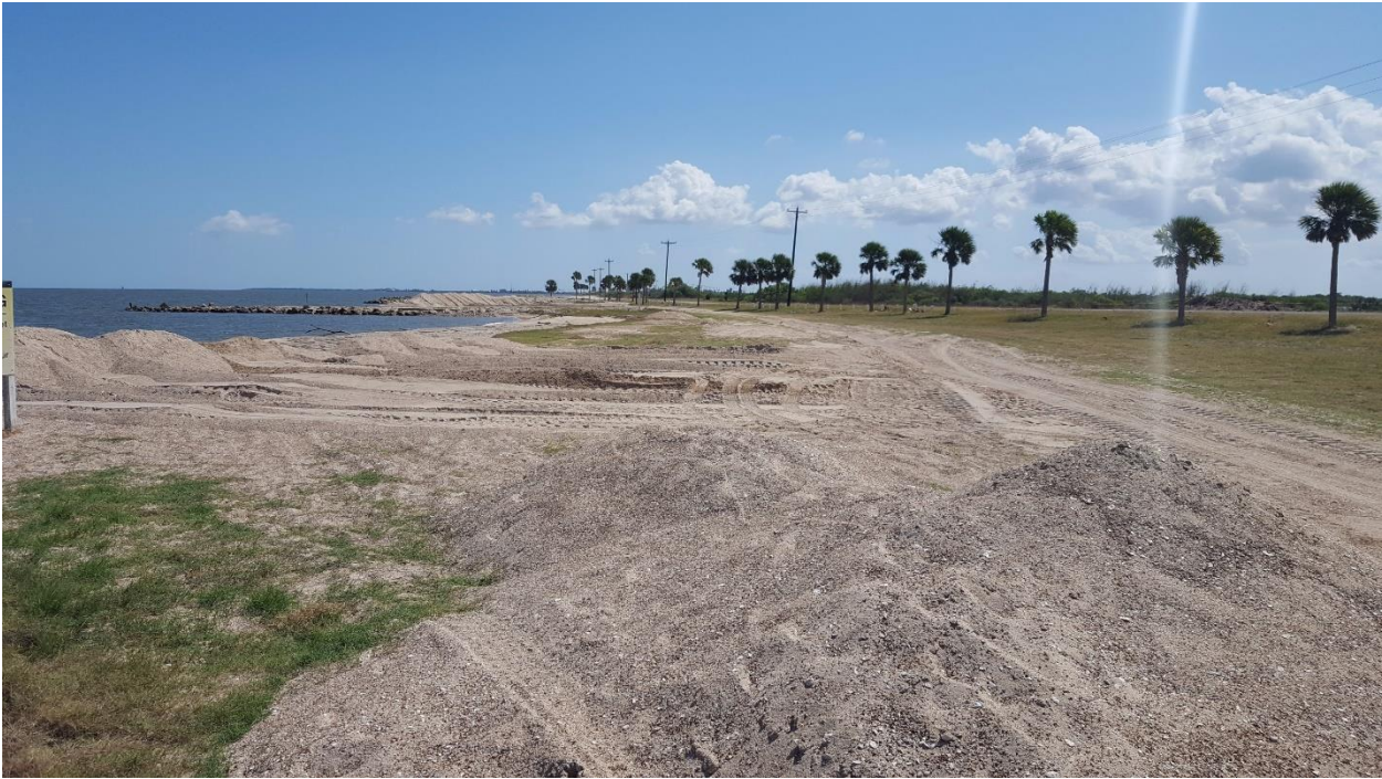
Southeast of STA 44+00
