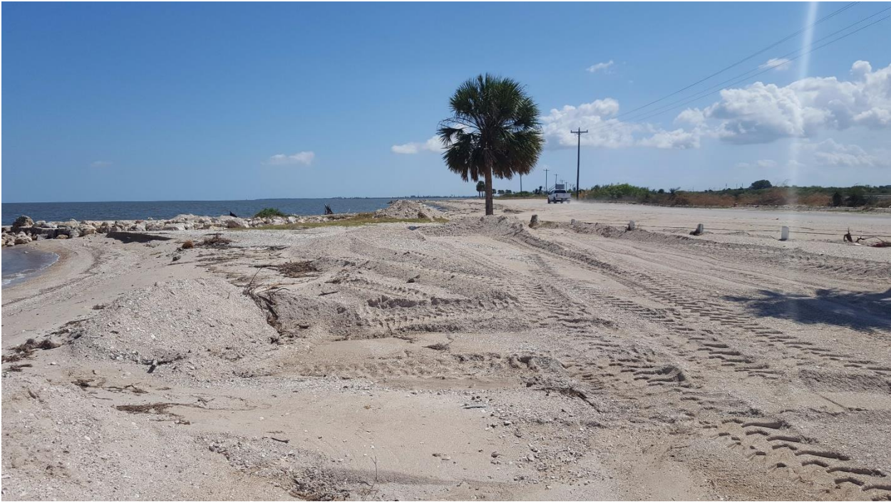
Southeast of STA 35+00
