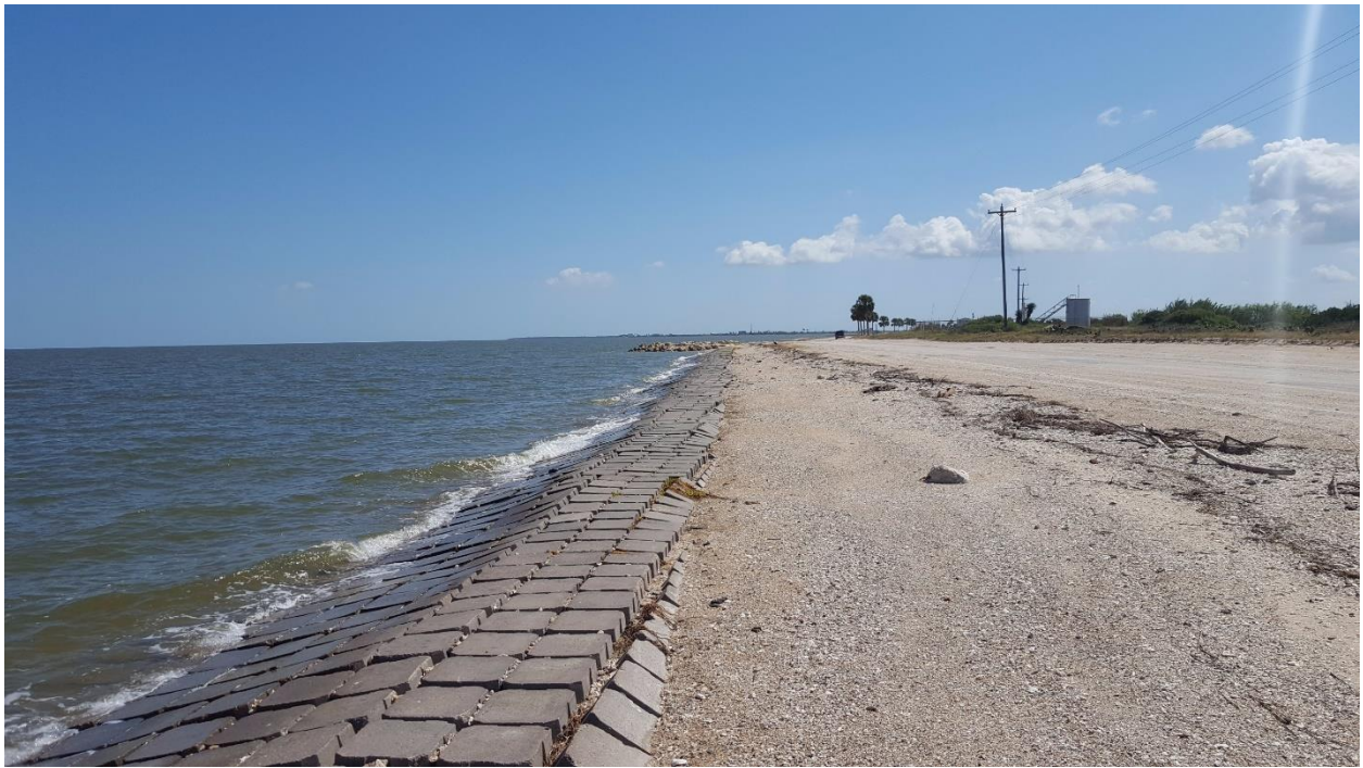
Southeast of STA 31+00
