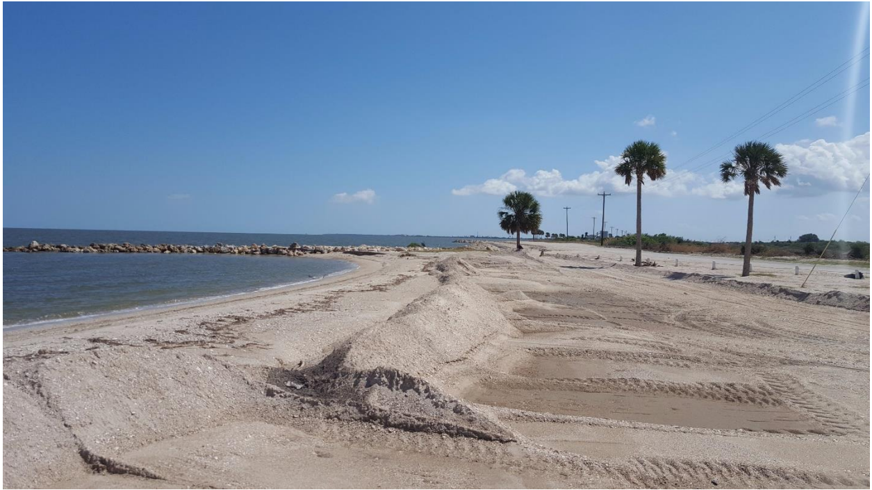
Southeast of STA 36+00
