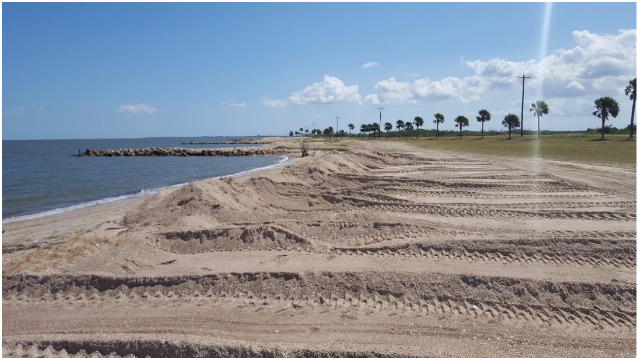
Southeast of STA 45 +80
