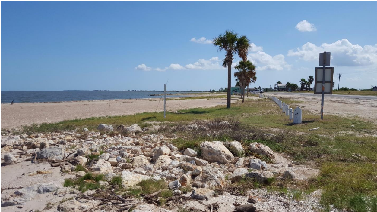
Southeast of STA 11+00
