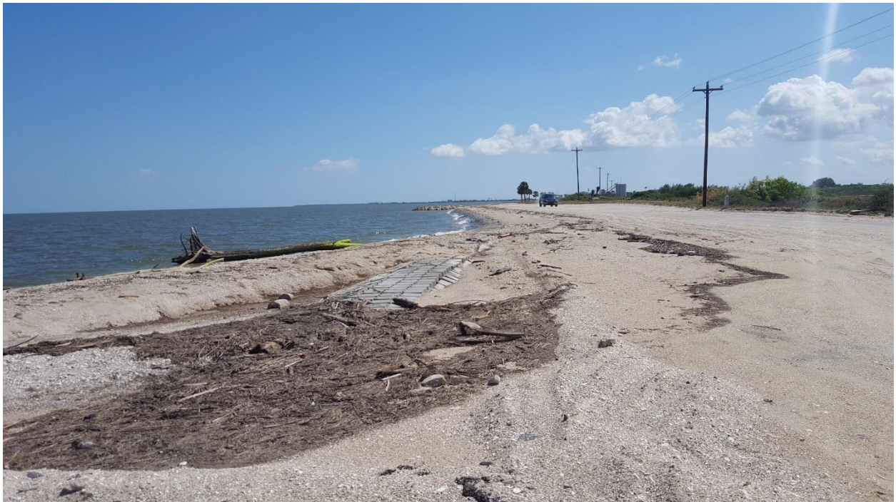
Southwest of STA 33+70
