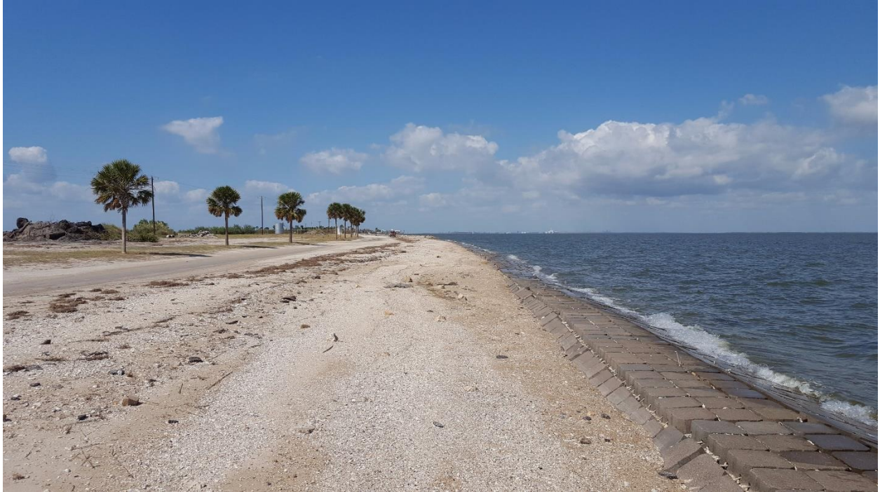
Northwest of STA 17+00
