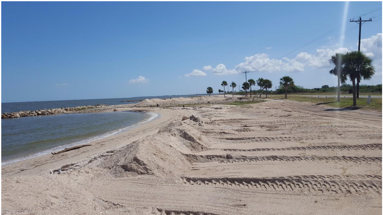
Southeast of STA 39+00
