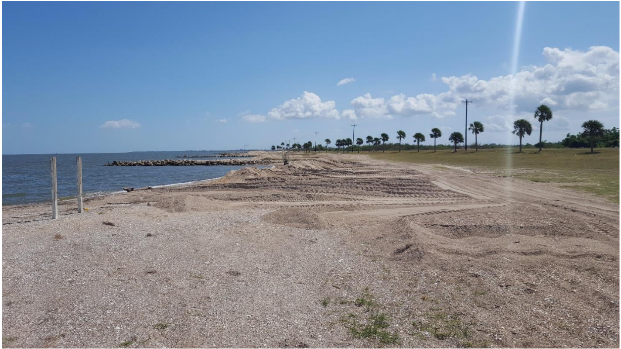
Southeast of STA 46+30
