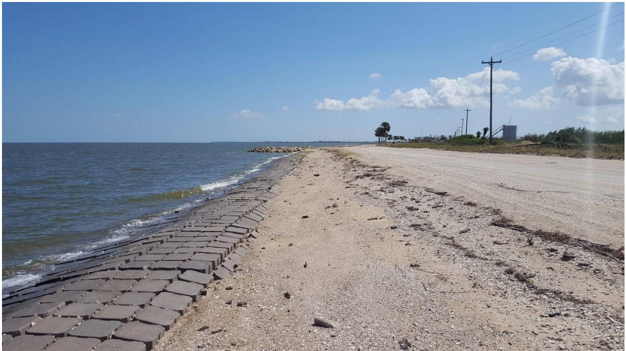
Southeast of STA 29+00
