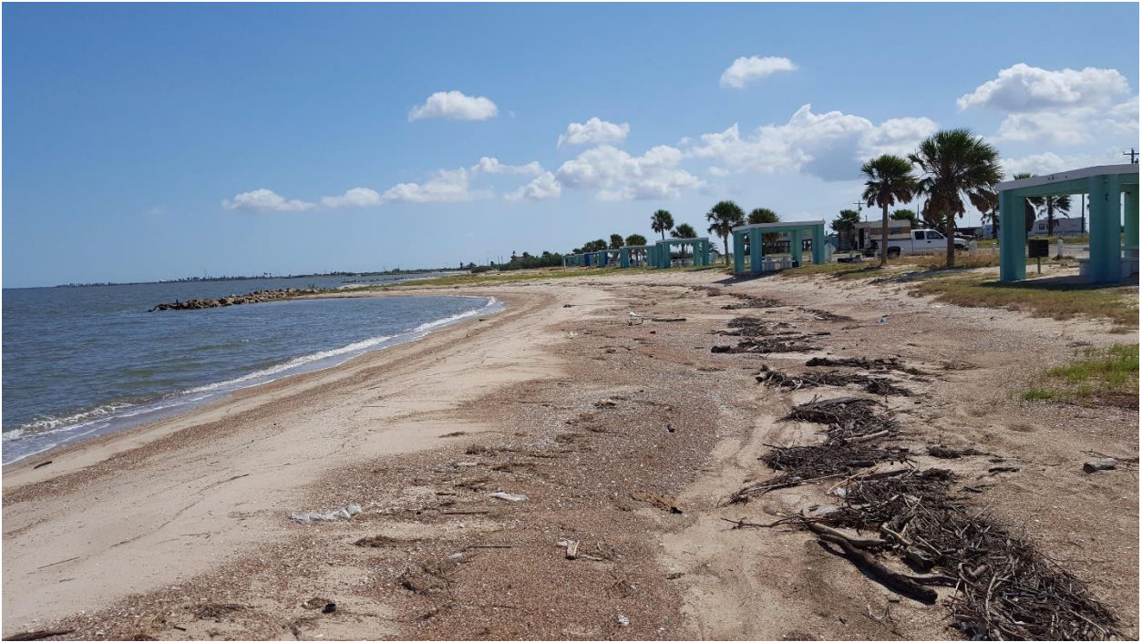
Southeast of STA 9+00
