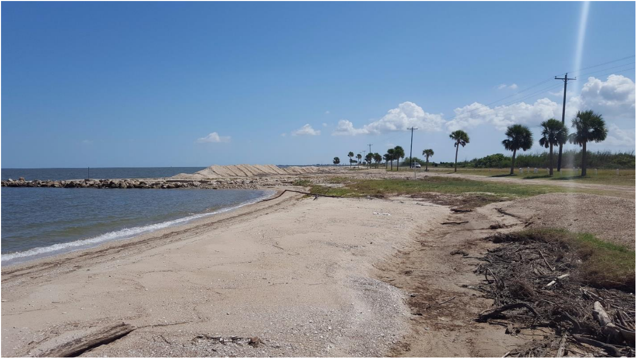
Southeast of STA 42+00
