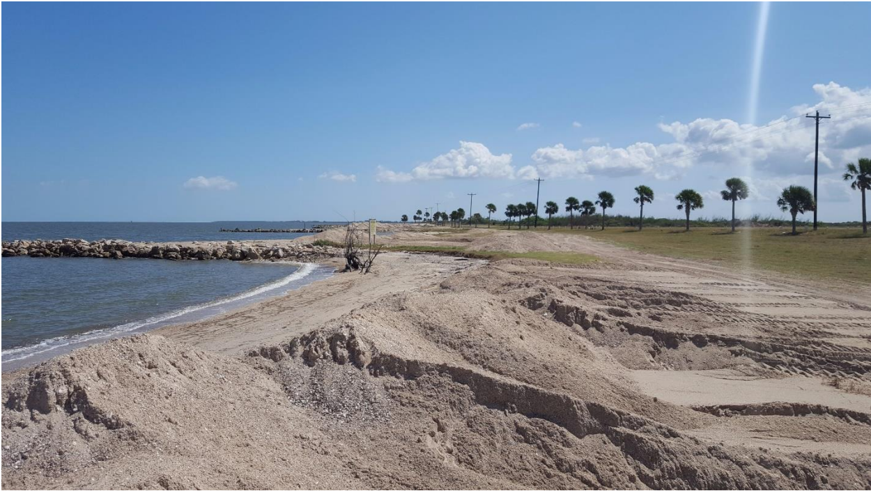
Southeast of STA 45+00
