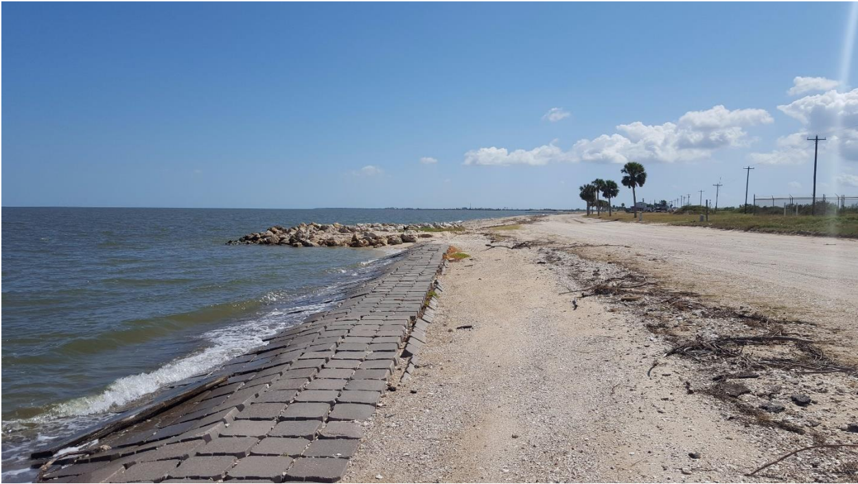
Southeast of STA 27+00
